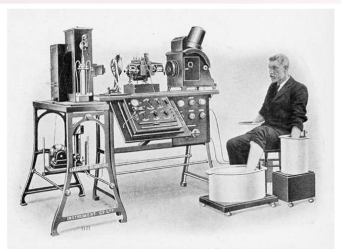
PHOTOGRAPH OF A COMPLETE ELECTROCARDIOGRAPH, SHOWING THE MANNER IN WHICH THE ELECTRODES ARE ATTACHED TO THE PATIENT, IN THIS CASE THE HANDS AND ONE FOOT BEING IMMEESED IN JARS OF SALT SOLUTION
